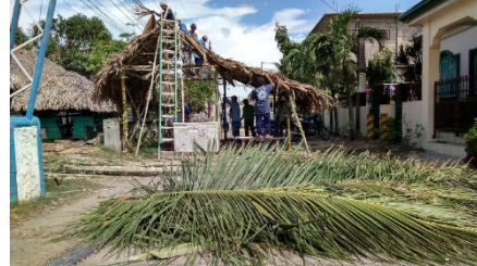
Figure 10. Coconut leaves were used in the roofing.
