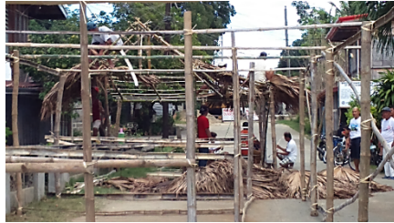
Figure 9. Bamboos were used for the construction of the hut.
